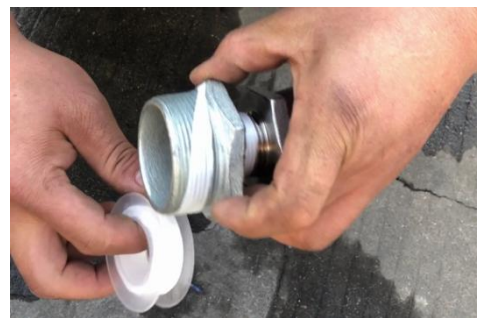
Step 4 Seal Reducing Joint with sealing tape.
