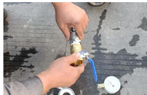
Step 3 Ball Valve connect to Tee Coupling, seal with sealing tape.
