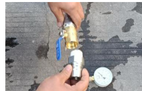
Step 4 Quick Connector A connect Ball Valve, seal with sealing tape.
