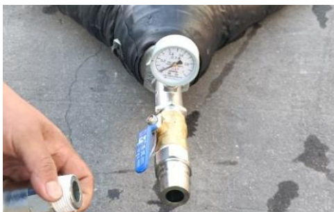
Step 5 Install Pressure Gauge to Tee Coupling.
