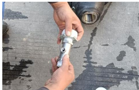
Step 2 Reducing Joint connect Tee Coupling, seal with sealing tape.
